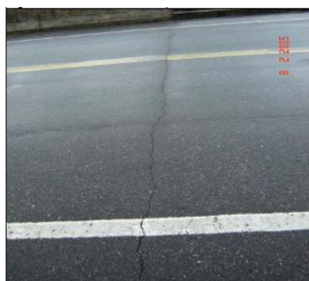
**Figura 08:** Fisura transversal
